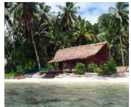
Figure 6. Completed bungalows at Wilderness Lodge, Solomon Islands
