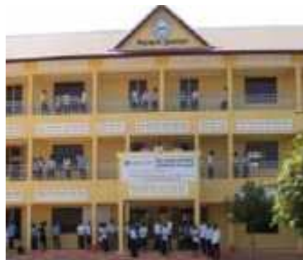
Figure 5. Bright Hope Institute new classroom building in Kampong Chhnang Cambodia
