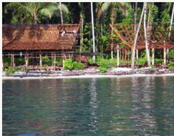
Figure 11. Bungalows under construction. Wilderness Lodge (Solomon Islands)
